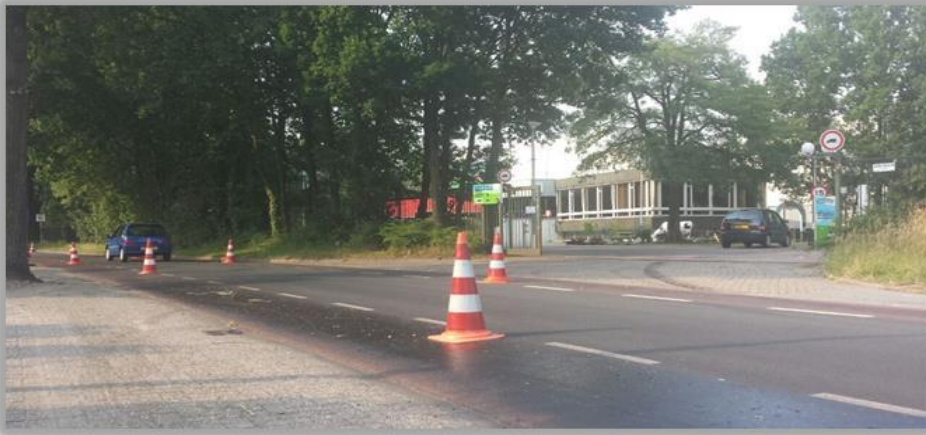
AFB. SMELTEND ASFALT (BRON: RTVOOST.INFO)
